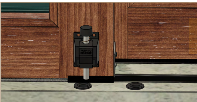
View of the left sash
